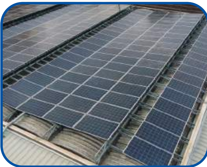
MCI ha installato 300 KW di impianto fotovoltaico MCI has installed 300 KW of photovoltaic system
